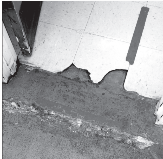
FIGURE 6–6 BROWNFIELD ISD KITCHEN FLOORING DECEMBER 2019
